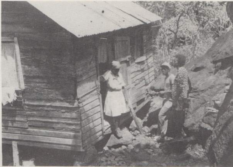
Coordinators of house repair program visit home to be repaired
